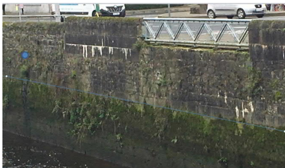
Photograph 16.1. View south of Charlotte's Quay. New outfall to be installed in the vicinity of existing outfall (blue dot), significantly above the typical flood level containing bryophytes, and indicated by a blue line.
