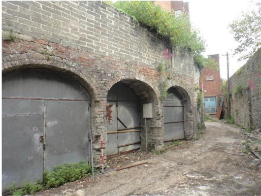
Plate 17.3 Internal lane to rear of building, facing northeast to Rutland St.
