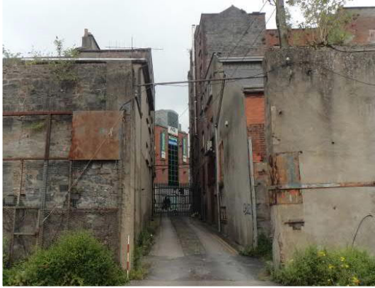
Plate 17.1 Laneway from internal courtyard,
