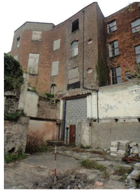
Plate 17.4 Rear of buildings fronting onto Patrick St., facing west
